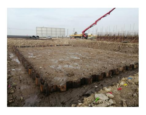
Lianyungang Petrochemical Co., Ltd is located in one of the seven National-Level Petrochemical Industrial Bases – XuWei District, Lianyungang Port, Jiangsu Province. The company is constructing a light hydrocarbon comprehensive processing and utilization plant with a performance of 3.2 million Mt/y. The sheet piles were used for the foundation works.
